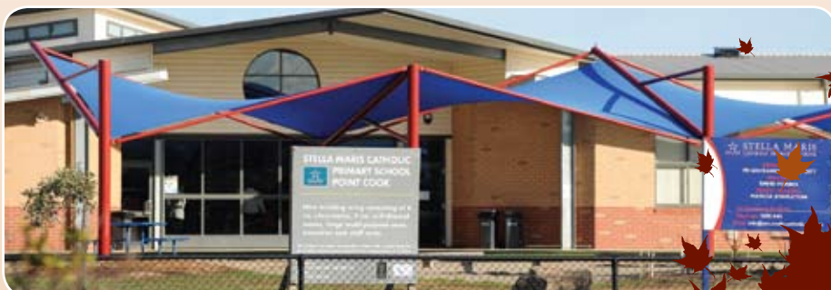
To accommodate the growing number of students, a new wing has been constructed at Stella Maris Catholic Primary School.
